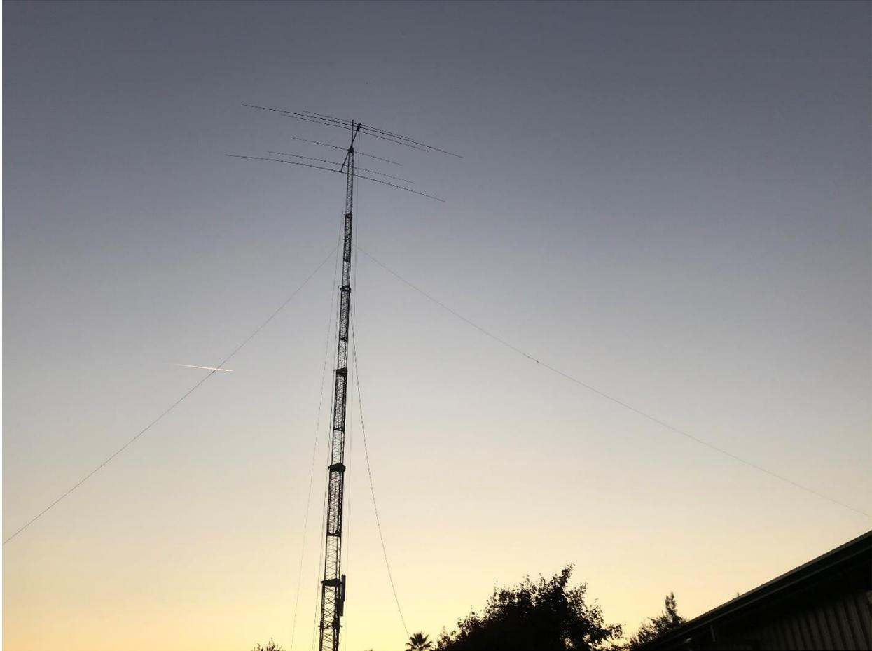
*Figure 5.* CQP 2019: NS6T antennas: 2-el Force12 C3S Yagi at 100ft., 40m Inv-Vee at 85ft., 80m Inv-Vee at 70ft. All supported by a US Tower portable tower trailer.
